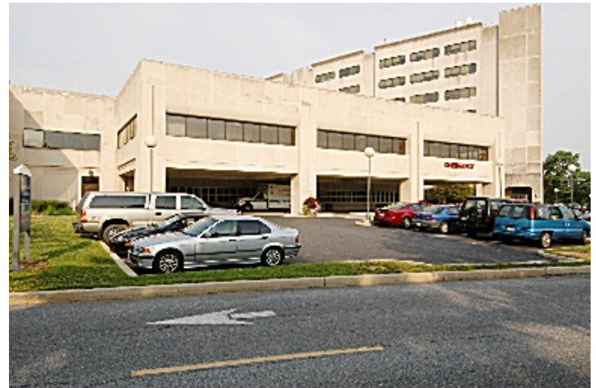
Fig. 3- Future ED Main Entrance
